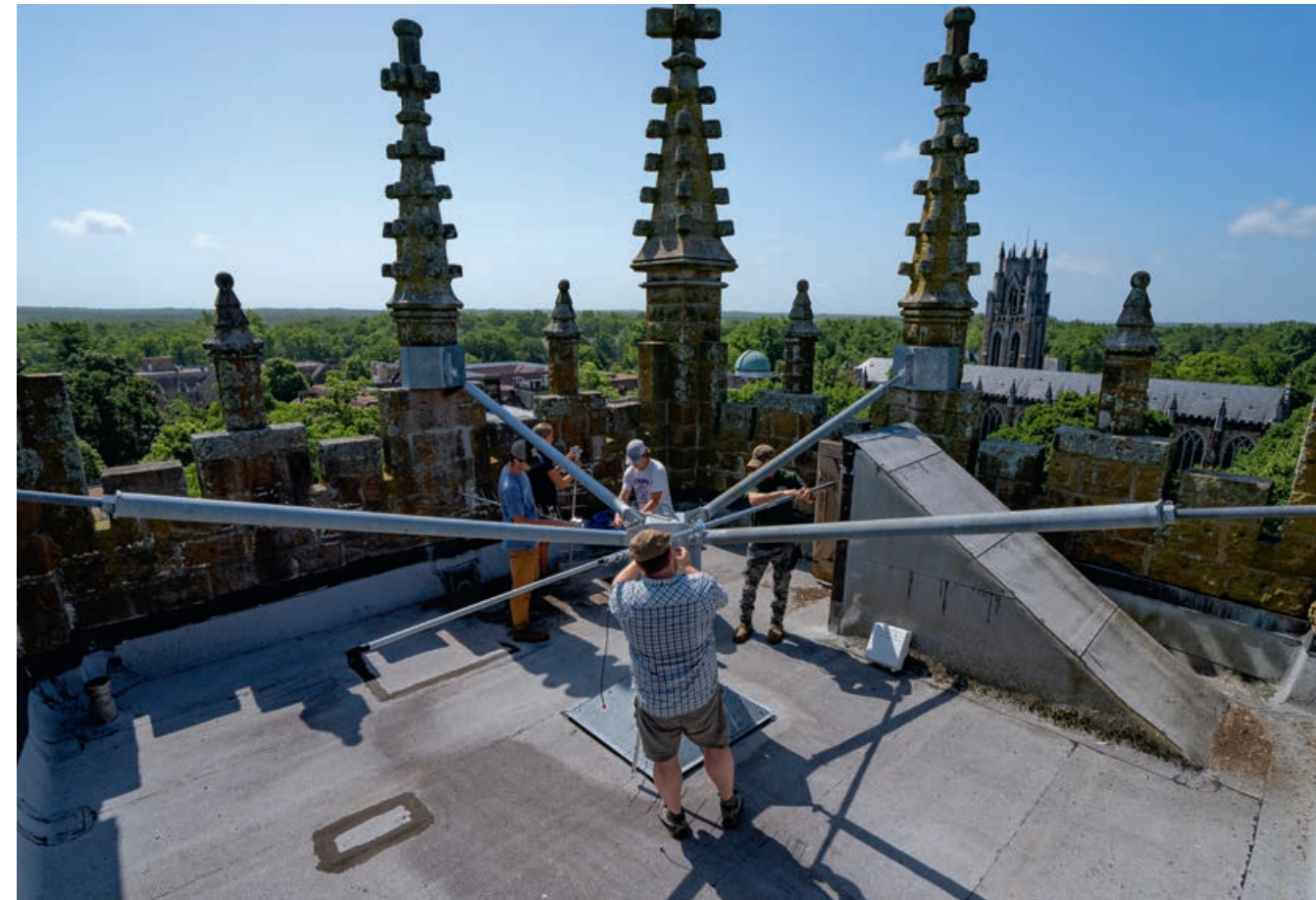
LISTENING: Holliday directs the installation of a Motus wildlife tracking receiver on the top of Breslin Tower at Sewanee: The University of the South.
