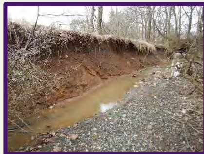
Stream restoration will address the steep, eroding banks at the Adduci project in the Rappahannock basin. (c) Wildlands Engineering
