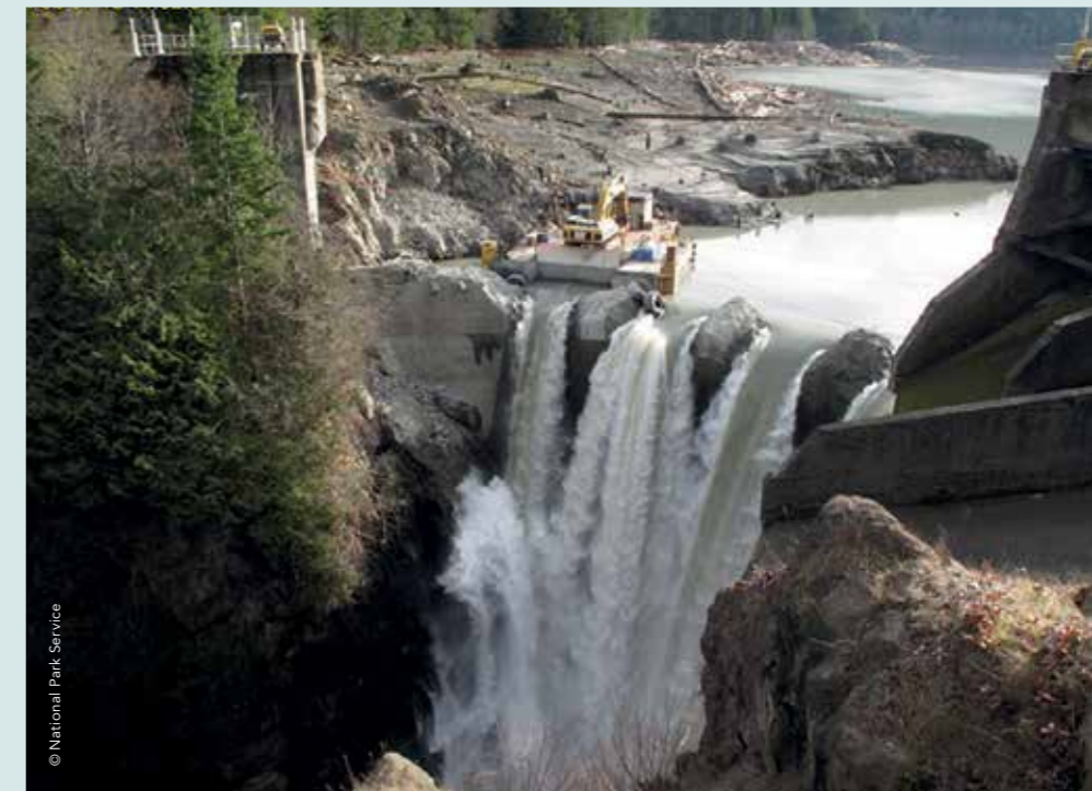
Removal of the Glines Canyon Dam on the Elwha River in 2014 (Washington state, USA), two years after removal of the Elwha Dam. These dams had caused a 99 percent reduction in the Elwha's salmon numbers, previously upwards of 400,000 per year across five species of salmon. The combined capacity of the two dams was 28 MW; since dam removal began, Washington State has added nearly 1000 MW of wind power.
