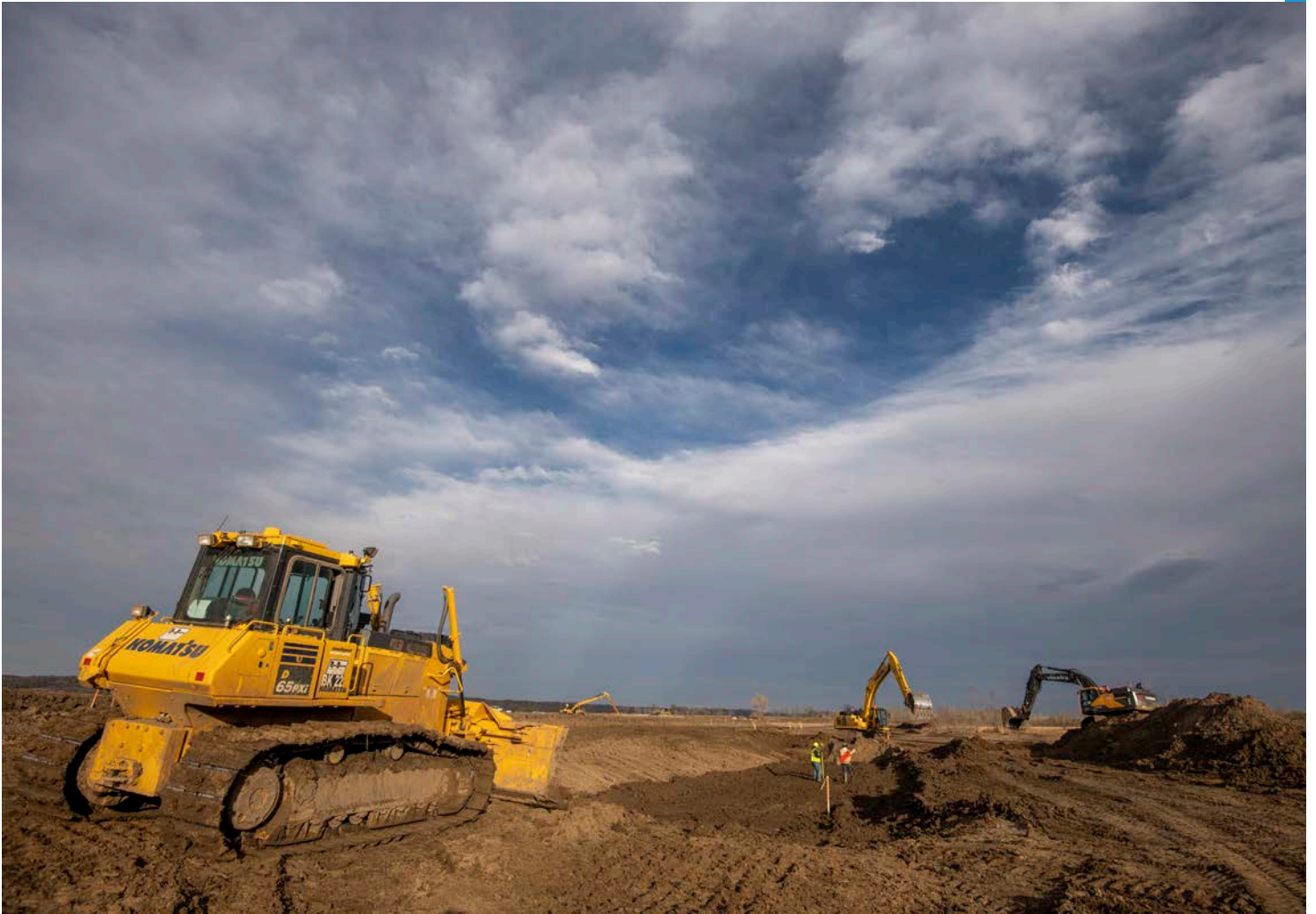
Crews conduct excavation work on the L-536 setback project, October 2020.
