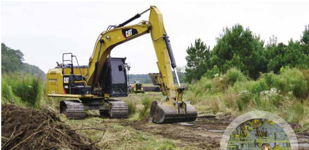
Heavy equipment is used to reshape an old farm field in the Pocomoke River headwaters to a landscape that more closely resembles a natural wetland. © Matt Kane/TNC; INSET Waterfowl, like wood ducks, are already benefiting from the restored habitat. © Deb Felmeij
